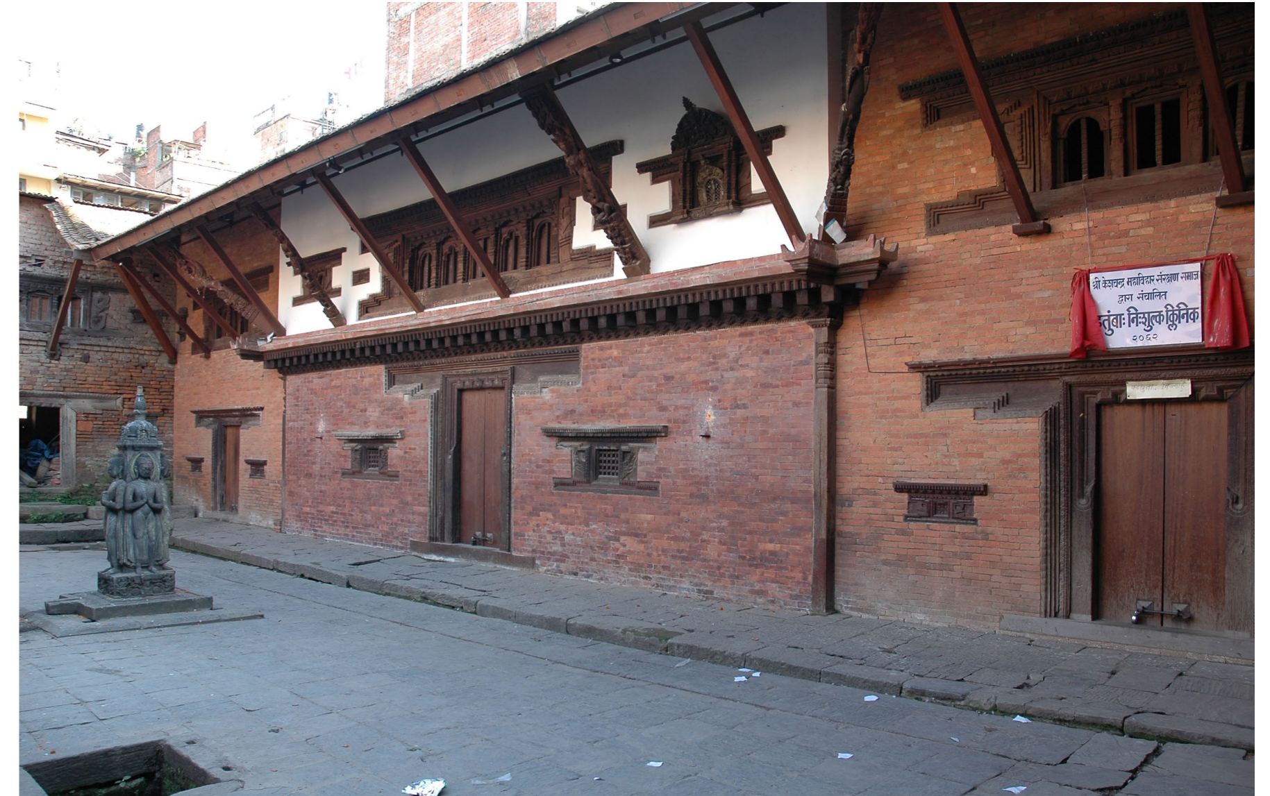
South wing courtyard elevation after restoration | November 5, 2006
