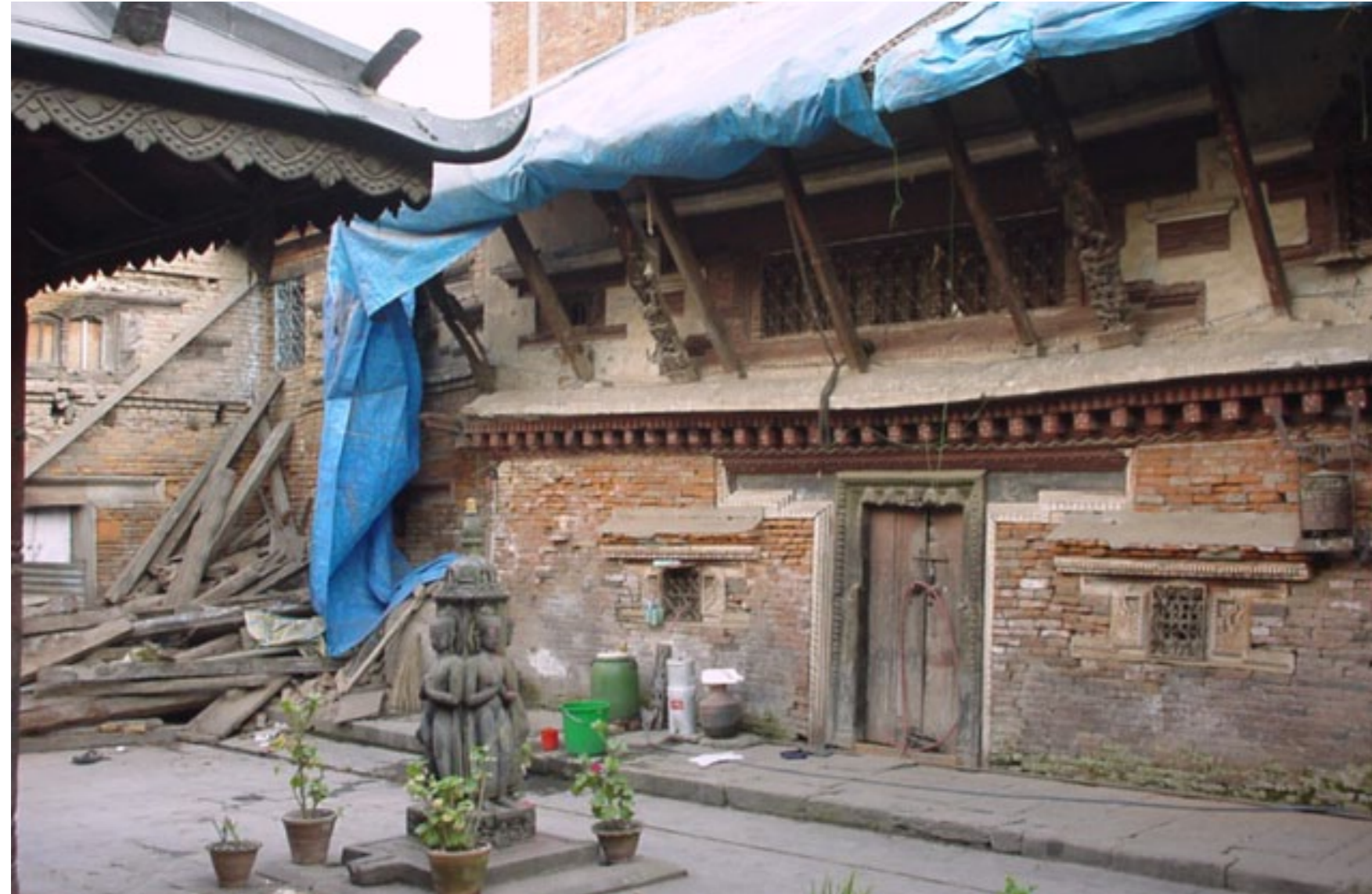
South wing courtyard elevation before restoration | March 20, 2000
