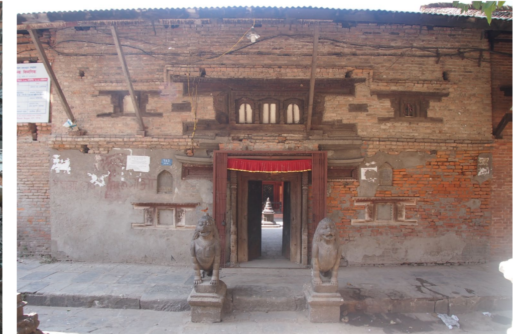
East wing, main entrance, existing conditions | 2012
