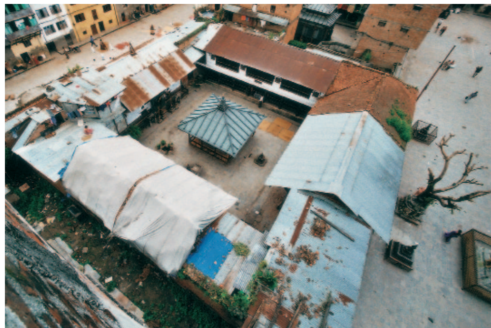
Itumbaha monastery | Nov 2002 When the restoration of Itumbaha was first proposed in 2002 only a small portion of the roof in the North-East corner still retained its historic mud and terracotta cover. All other historic roofs had been lost and were rebuilt employing corrugated steel sheets. The shapes of the roofs had been significantly changed: note the shed roofs in the foreground and the addition of a projecting balcony as seen on the south-west corner of the building.
