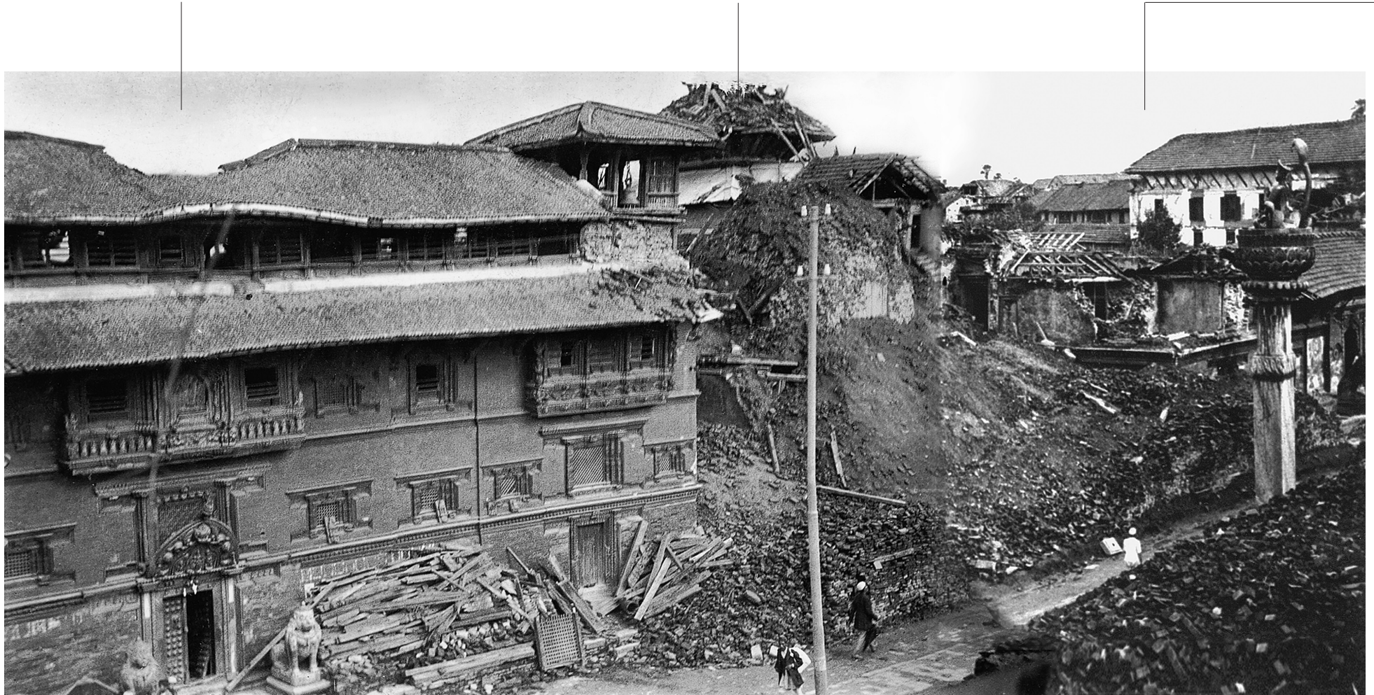
Patan Darbar after the earthquake | View from the Northwest, 1934 This photograph shows the extent and type of damage after the 1934 Bihar-Nepal earthquake. The collapse of the four “floating” Taleju temples caused extensive damage to the relatively stable courtyard buildings upon which they stood.
