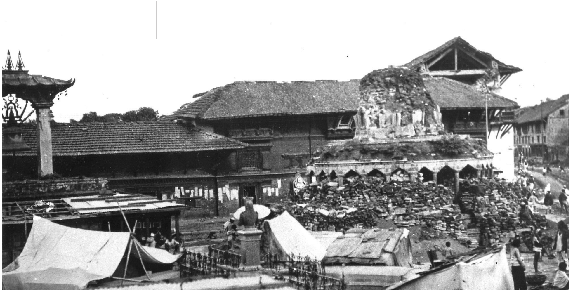
Patan Darbar after the earthquake | View from the West, 1934 Three of the four temples were rebuilt in 1935-1938 using mostly salvaged materials collected from the rubble. Since the reconstruction occurred
