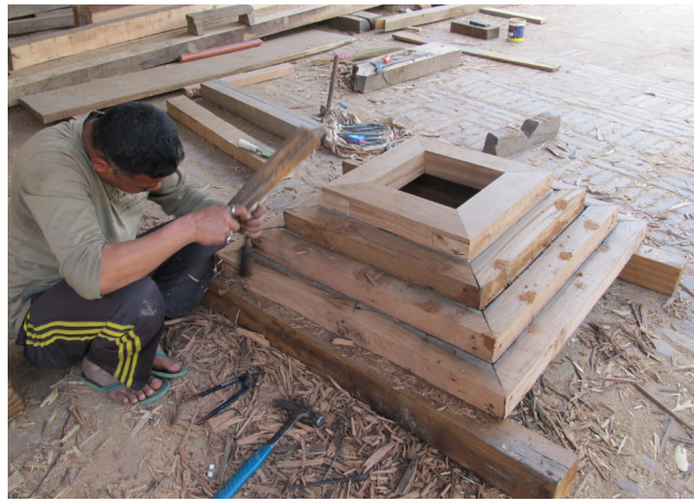
Reconstruction of timber structure | April 2014 Carpenters constructed a new timber structure for the stepped plinth of the miniature sikhara temple on the pinnacle.
