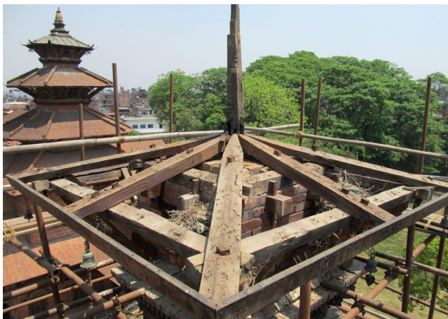
Removal of common rafters | April 22, 2014
