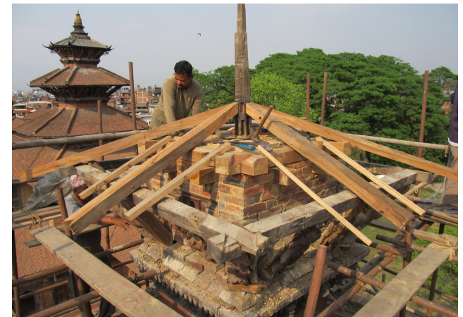
Assembly of central and corner rafters | April 28, 2014 The central and corner rafters (sal wood) were placed in an alternating sequence before assembly of the common rafters (pine).
