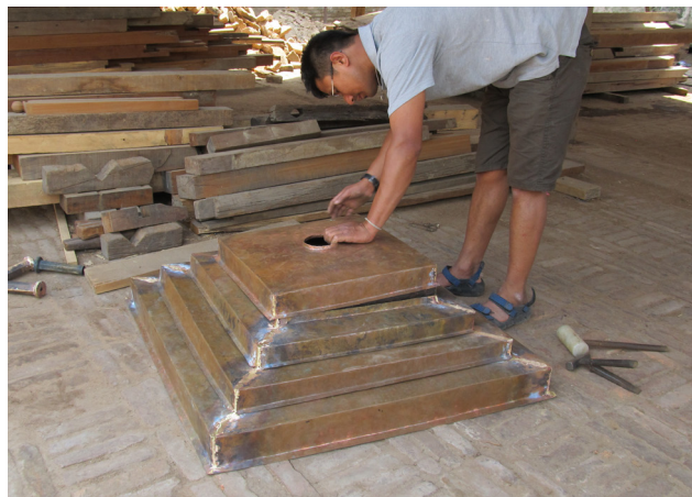
Reconstruction of timber structure | April 2014 Carpenters constructed a new timber structure for the stepped plinth of the miniature sikhara temple on the pinnacle.
