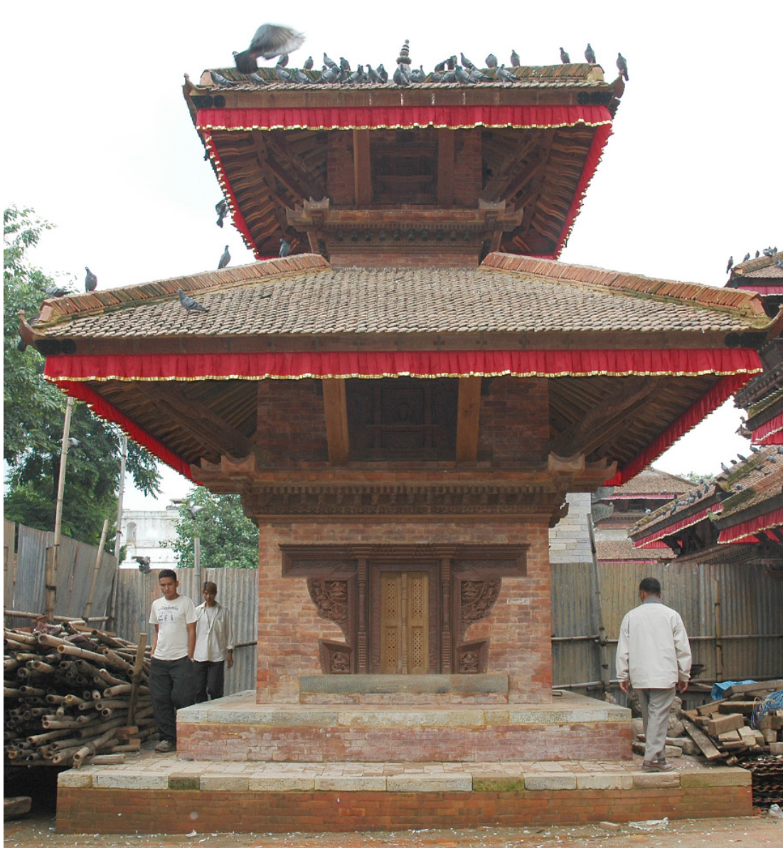
top left: The plinth was constructed with traditional dachi appa brick in mud yellow mortar. Dressed stone apron encircles the plinth on top and is paved with traditional telia tiles. Photo by: Lumanti Joshi, June 2007.
