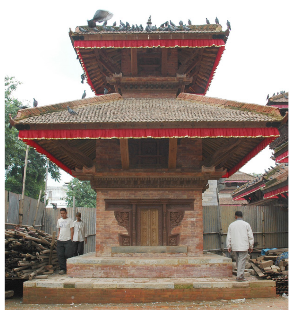
right: Lakshmi Narayan Temple, 2007. The entire structure was recreated with the help historical photographs. After a detail study of elements from similar temples of the same time period, carving details such as the doors, windows and the cornices were carved. Photo by: Lumanti Joshi, August 2007.
