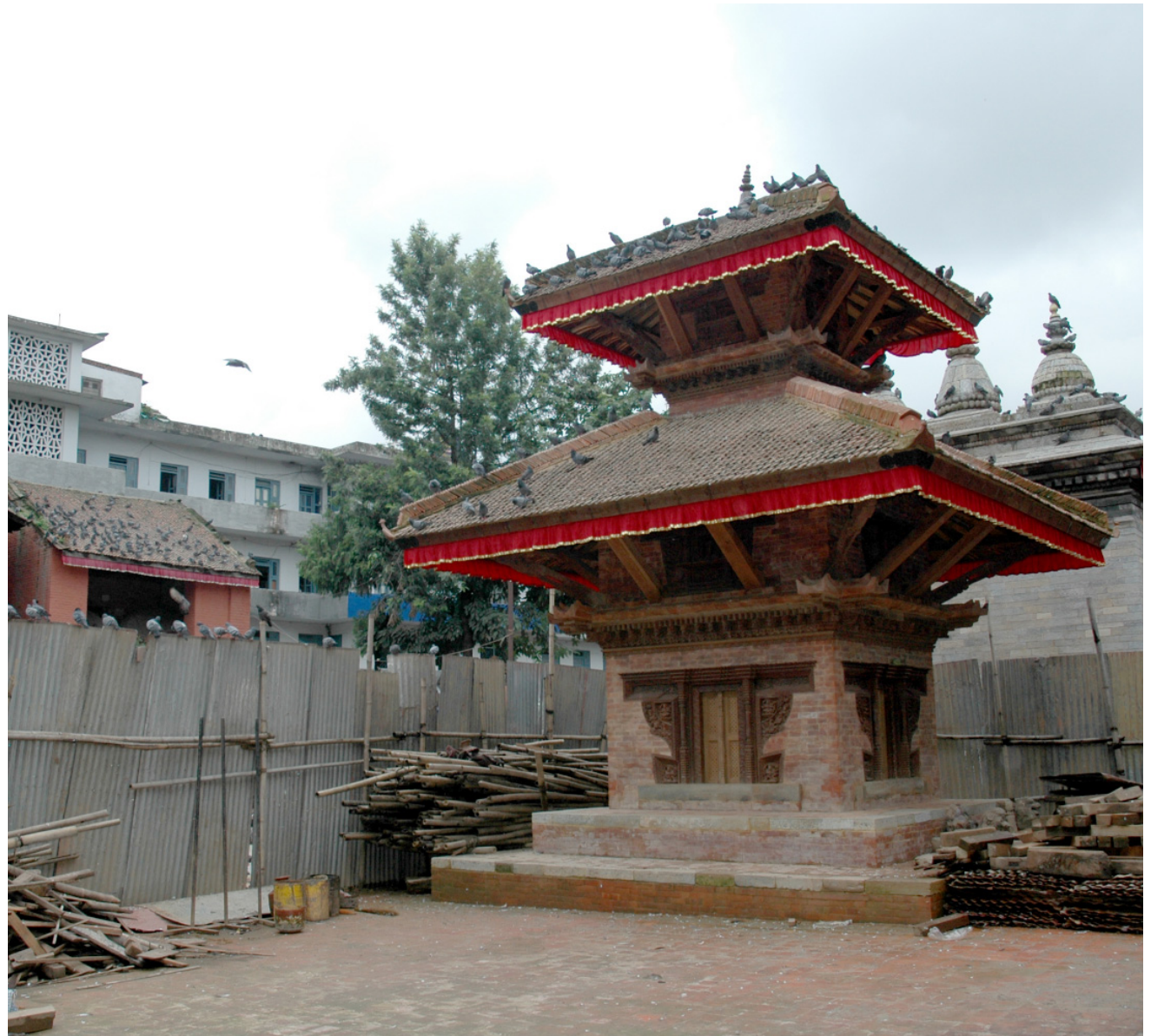
right: When the carving of the corner struts were complete, these were tried out in their respective positions for their precise size. Sometimes carpenters had to make minor correction for readjusting them. Photo by: Lumanti Joshi, June 2007.
