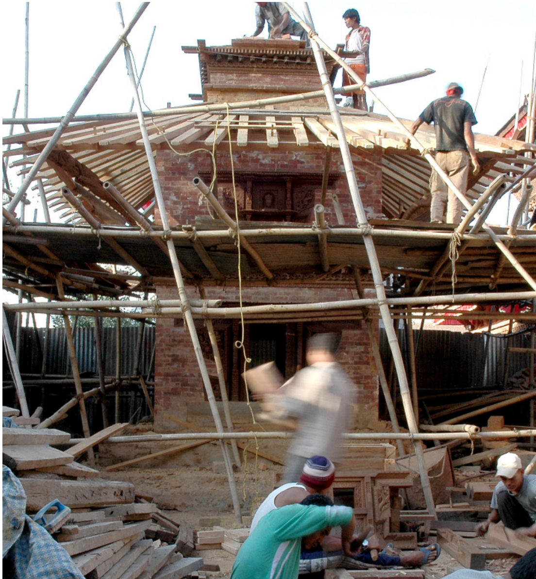
top: The corner struts from the Mahadev Temple I, where the restoration work had simultaneously begun, were used as a base for recarving the ones for this temple. Photo by: Lumanti Joshi, November 2006.
