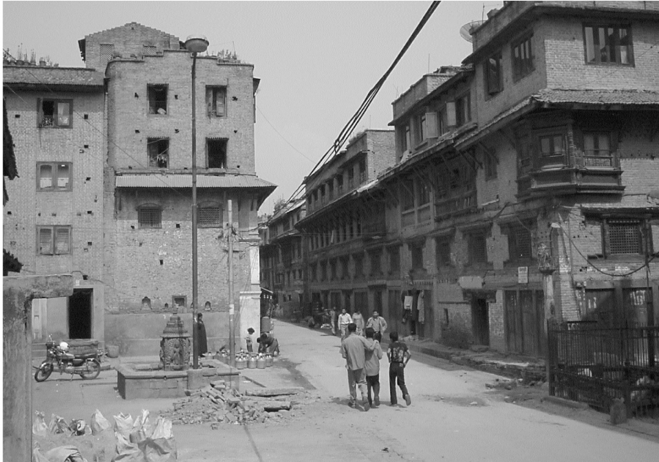
15. The area where the pati existed laid vacant before reconstruction.
