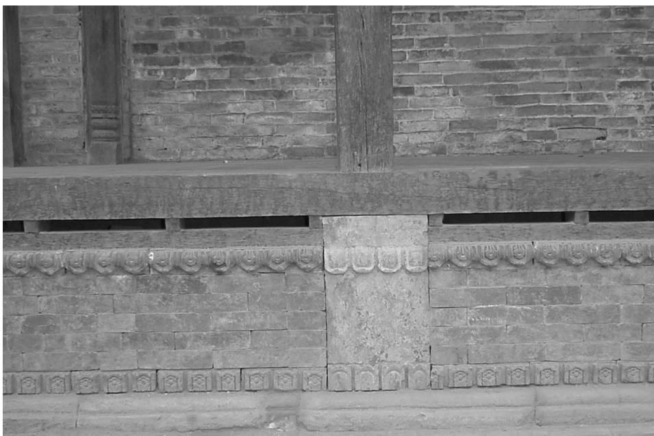
5. The plinth was reconstructed using traditional materials and technology.
