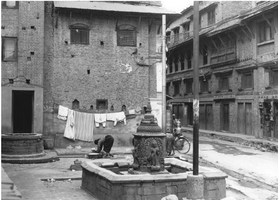
1. Chabaha pati was completely lost in the 1934 earthquake. Existence of the rest house was only visible on the wall of the adjacent residence, and from the old brick foundation.
