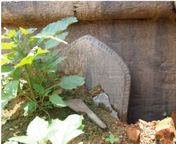
Stele on the northern lower plinth The inscription is partly obscured by debris. It should be brought to a safe storage area.
