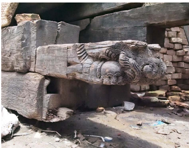
Beam end from the inner cella This beam is most likely part of the original 17th century temple and could possibly be reused in the reconstruction.
