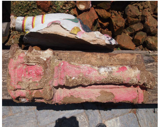
A column from one of the 12 terra cotta niches Heavy layers of lime and enamel paint obscure this terra cotta fragment which makes identification of the figure impossible.
