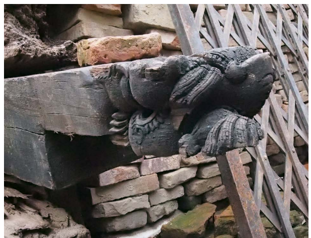
Beam end from the inner cella This beam is most likely part of the original 17th century temple and could possibly be reused in the reconstruction.
