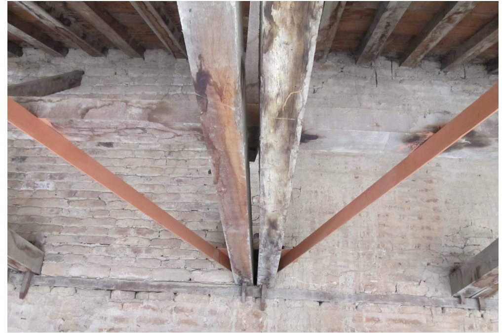
Details of steel cross-bracing of gallery level roof | October 2012
