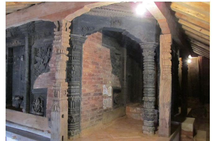
Southeast corner of the inner sanctum after rehabilitation | October 2012 For the new roof support system historic carved columns were used. To compensate for the room height, the columns were extended. These columns were strategically placed much closer to the inner structure for maximum support.
