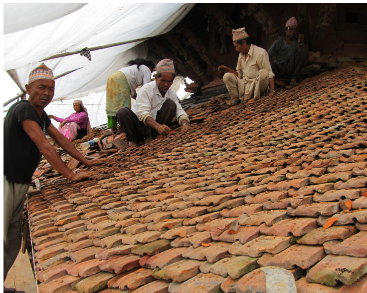
far left: The waterproof membrane is installed over the plyboard. This will protect the timber against any future water infiltration, and acts as a waterproof layer.
