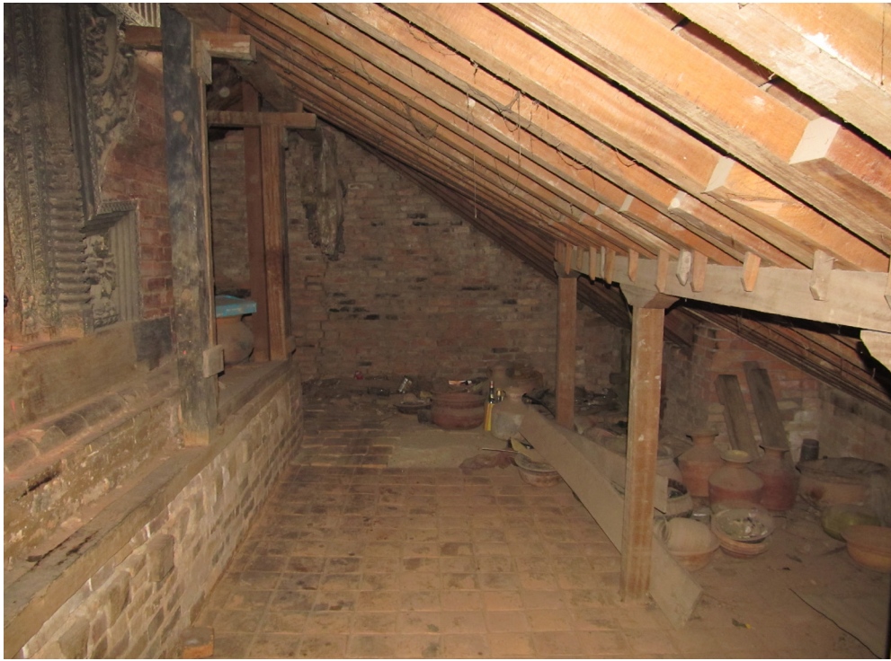
Roof before rebuilding | April 2012
