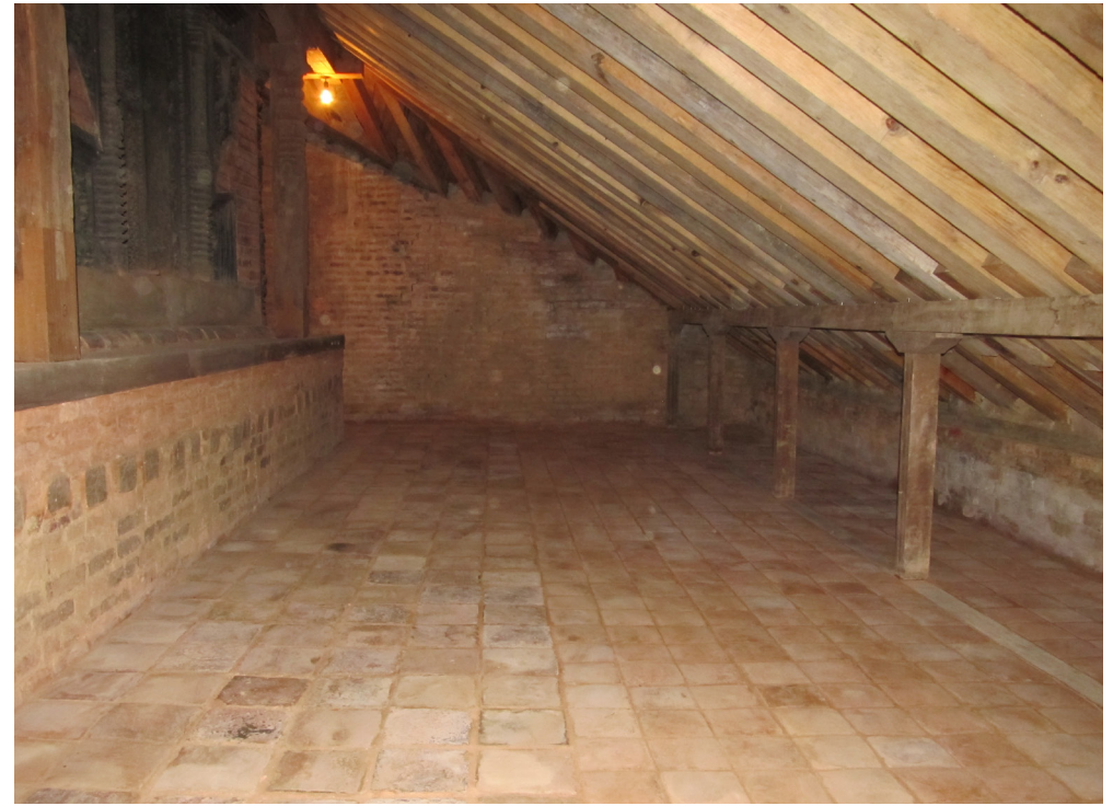
Roof after restoration | October 2012
