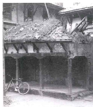
Kwalakhu Pati and Urban upgrading, Patan, 1993
