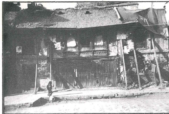
Ayuguthi Sattal Restoration Project: Ongoing with model funding from both the U.S. Andy Warhol Foundation and local businessman Himalaya Pande, this highly visible site on Patan's Darbar Square will encourage similar partnerships in the future. The government decision to nationalize the threatened structure, a landmark precedent, will be critical for hundreds of threatened "A-class" monuments in Nepal.
