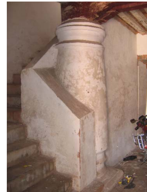
The main stair of the Court Building This unique pier marks the grand ascent to the upper floors. The original tile treads and risers were recently covered with Portland cement plaster.
