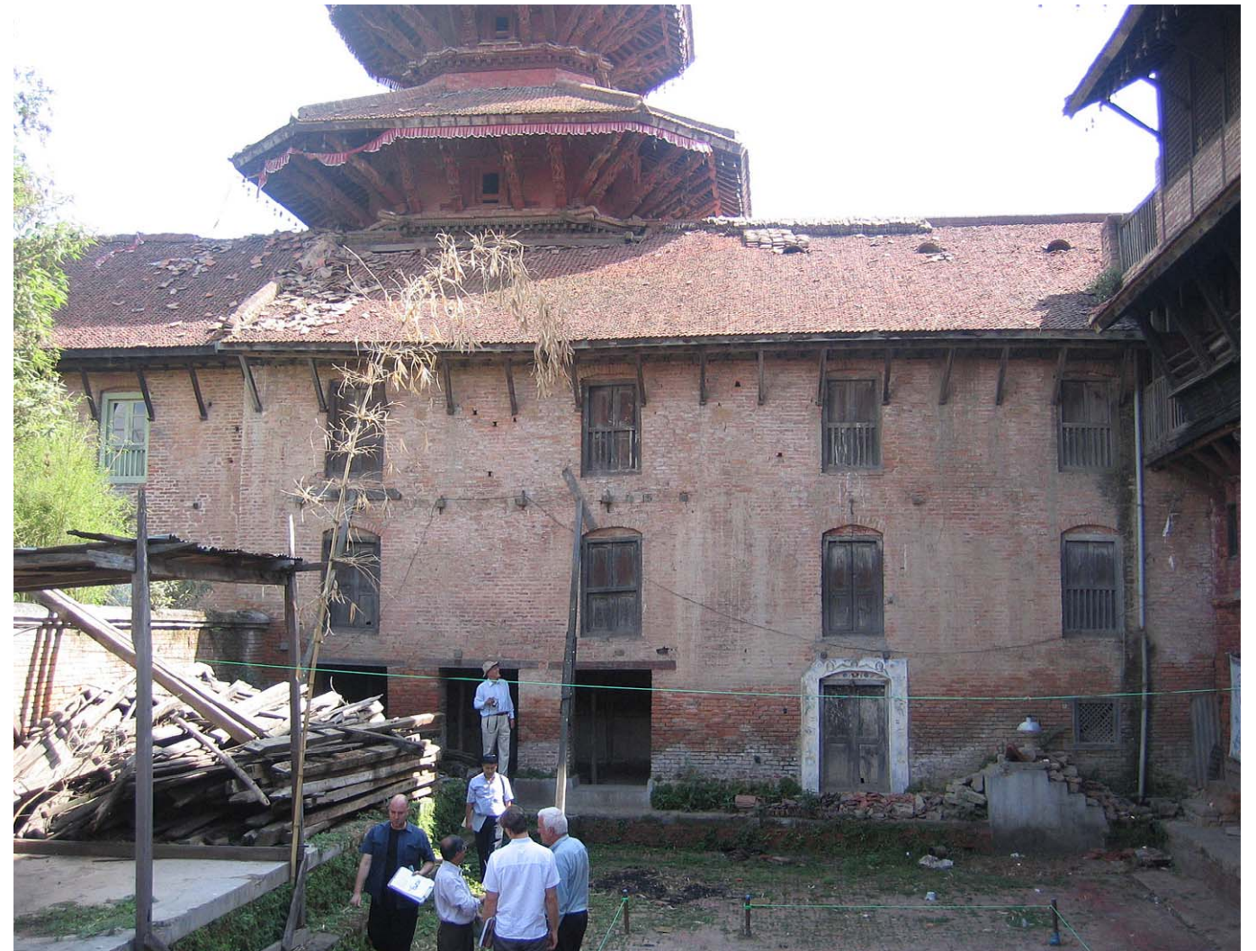
Nasal Cok looking south Assessment of roof is required to determine if reconstruction is recommended. Photograph, May, 2006
