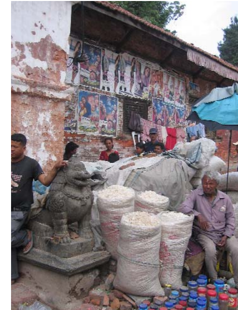
Salt traders at the entrance to the Court Building The presence of salt has caused extensive damage to the traditional lime-brick plaster finishes.
