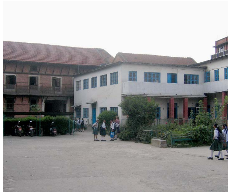
Object #02: extension of school building butting up against the 17th century shrine building and the North wing. A compromise could be found with the school to support construction of additional rooms in the main courtyard in exchange for demolishing this inappropriate structure.
