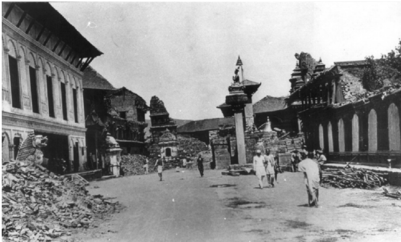
Bhaktapur Darbar Square Comparative views before and after the 1934 earthquake
