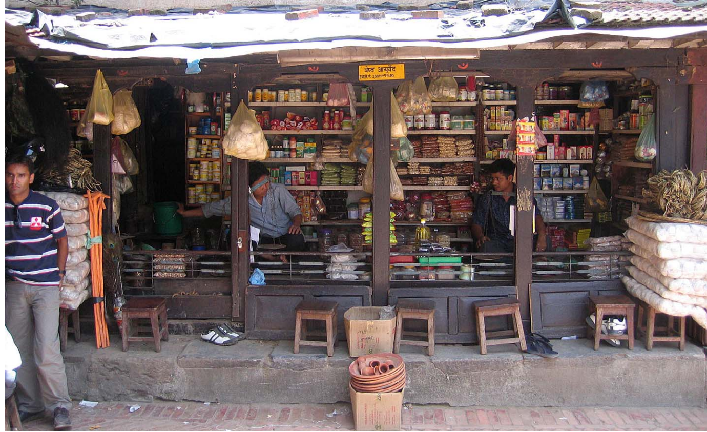
far left and left: Medicine shops in front of Sundari Cok and the Court Building Ever since the earliest photographic documentation available these small shops have been occupied by traders of Ayurvedic medicine and other food and household items. Adjacent lower and first floor rooms in Sundari Cok and the Court Building serve as storage rooms. The stalls' roofs are in poor condition and only a few carved timber elements remain from the 19th century. Photograph, 2006.
