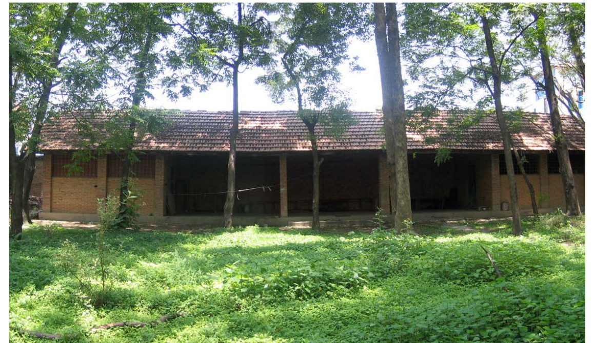
Object #04: storage shack for stone fragments and materials for Patan Museum garden maintenance
