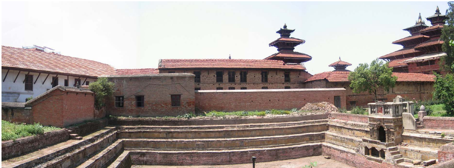
Demolition Objects # 11 and #12: The rear wall of the abandoned police post and the new Boundary wall behind the tank. Note the grade level around the tank which is now 4-5 feet higher than it was 150 years ago.
