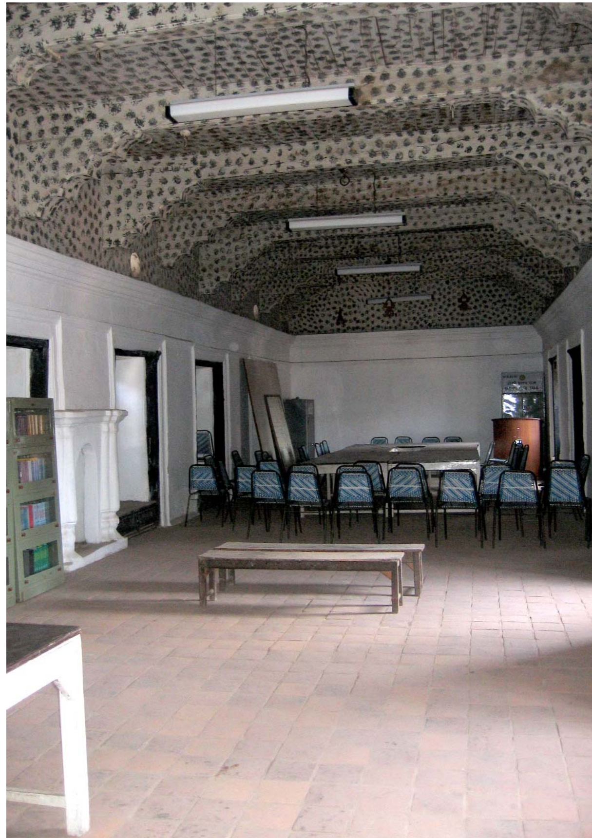
North Wing - main hall on the top floor This is the first building in Nepal featuring a room of more than 5 meters in width. The roof incorporates heavy timber trusses. Photograph, May, 2006
