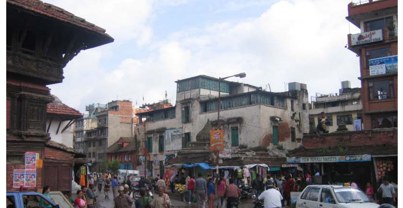
View of Demolition Object # 13 from Darbar Square The South-West corner of Sundari Cok on the left and a modern 7-story building on the right.
