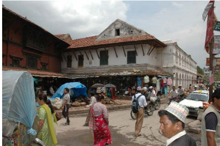
View looking east toward the Court Building Commercial encroachment at the south of Sundari Cok and the west of the Court Building. All photographs on this page: May, 2006
