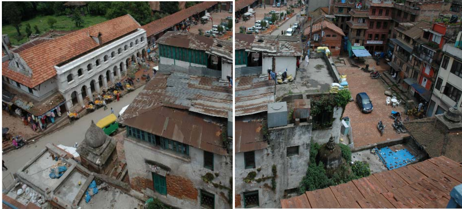
Birds eye view of Demolition Object # 13: Police Station To the left the Court Building, in the background garden and Kot pati
