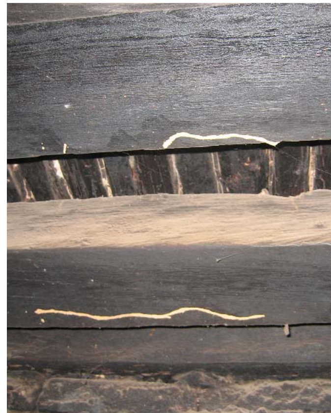
far left: Storage room on the first floor of Sundari Cok Parts of the courtyard's southern wing is used for storage by the medicine shops located in the southern shed. Photograph, 2006.
