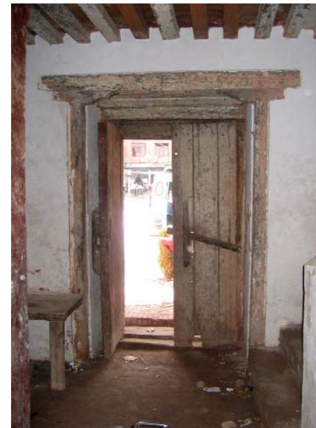
Interior view of the main entry The large scale of this doorway was a departure from the diminutive scale favored by traditional Newar builders. Note that the outside grade is higher than the threshold of the door.
