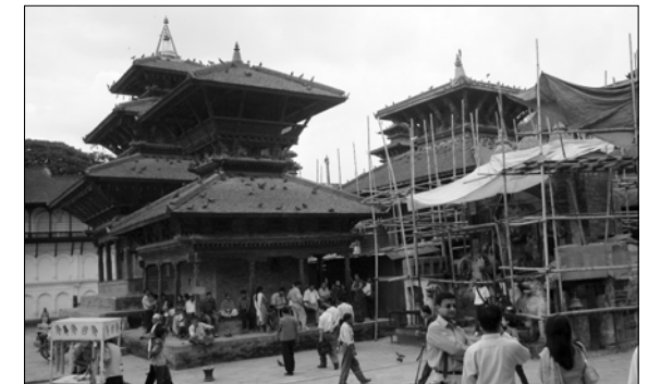
Similar view after the restoration of Indrapur (in foreground) and Narayan Temples. Photo: Raju Roka, June, 2004.
