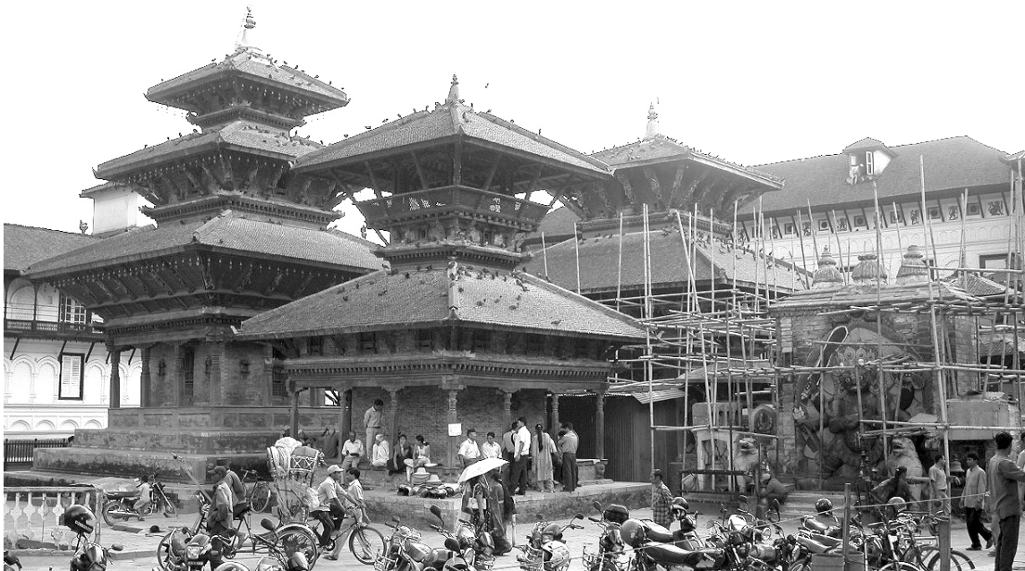
above: The temples at the Darbar Square before the “Kathmandu Darbar Initiative” project. Photo: Rohit Ranjitkar, June 1999.
