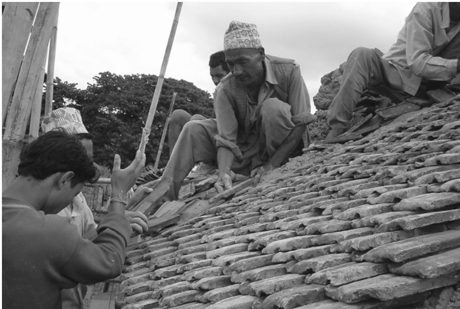
above: Carpenters fitting the wall plates incorporating the steel plates to stabilize the structure. Photo: Badri Juwal, July 2003.
