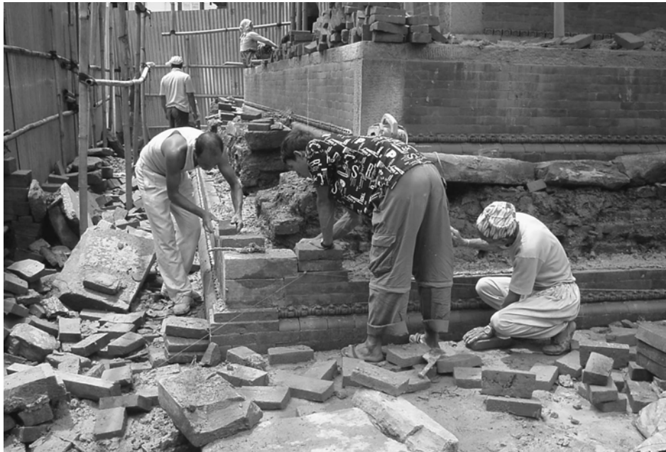
above: Preparation of mud, traditional material used for mortar for the construction. Photo: Raju Roka, September 2003
