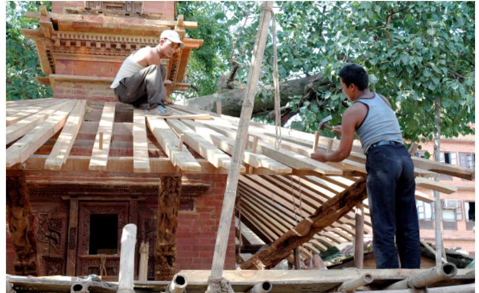
above: The carpenters installing timber roof structure in the lower level. Photo by: Lumanti Joshi, May 2007.
