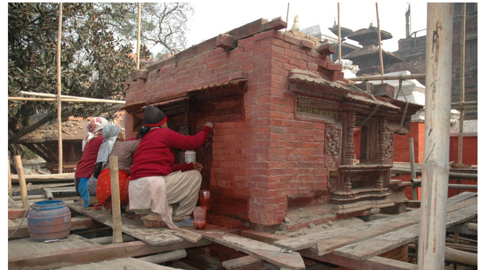
right below: The unsightly red paint from the carved elements were removed using soft brush and mild detergent. Photo by: Lumanti Joshi, March 2007.
