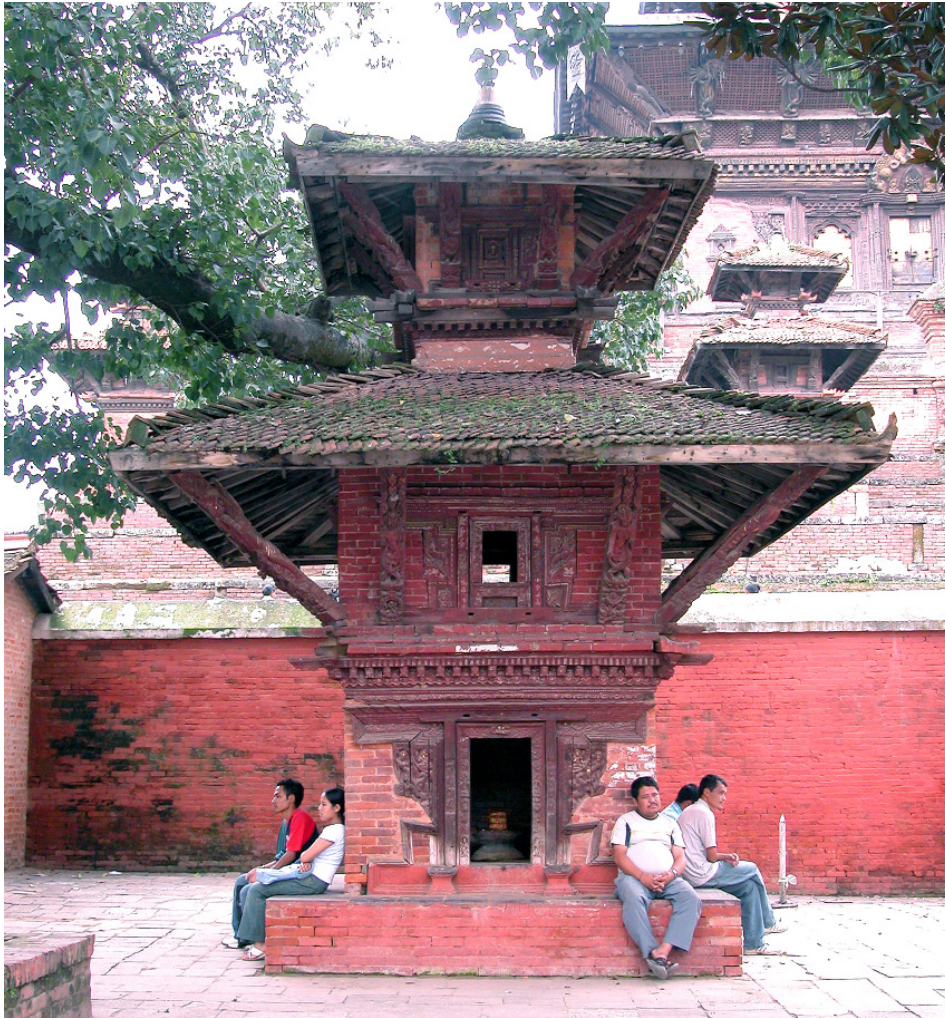
left: The Mahadev Temple I as it stood in December 2006. The roof structures were in poor state and in urgent need of repair. Photo by :Lumanti Joshi.
