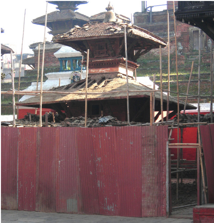
above: The roof structure being dismantled. Photo by: Raju Roka, February 2007.
