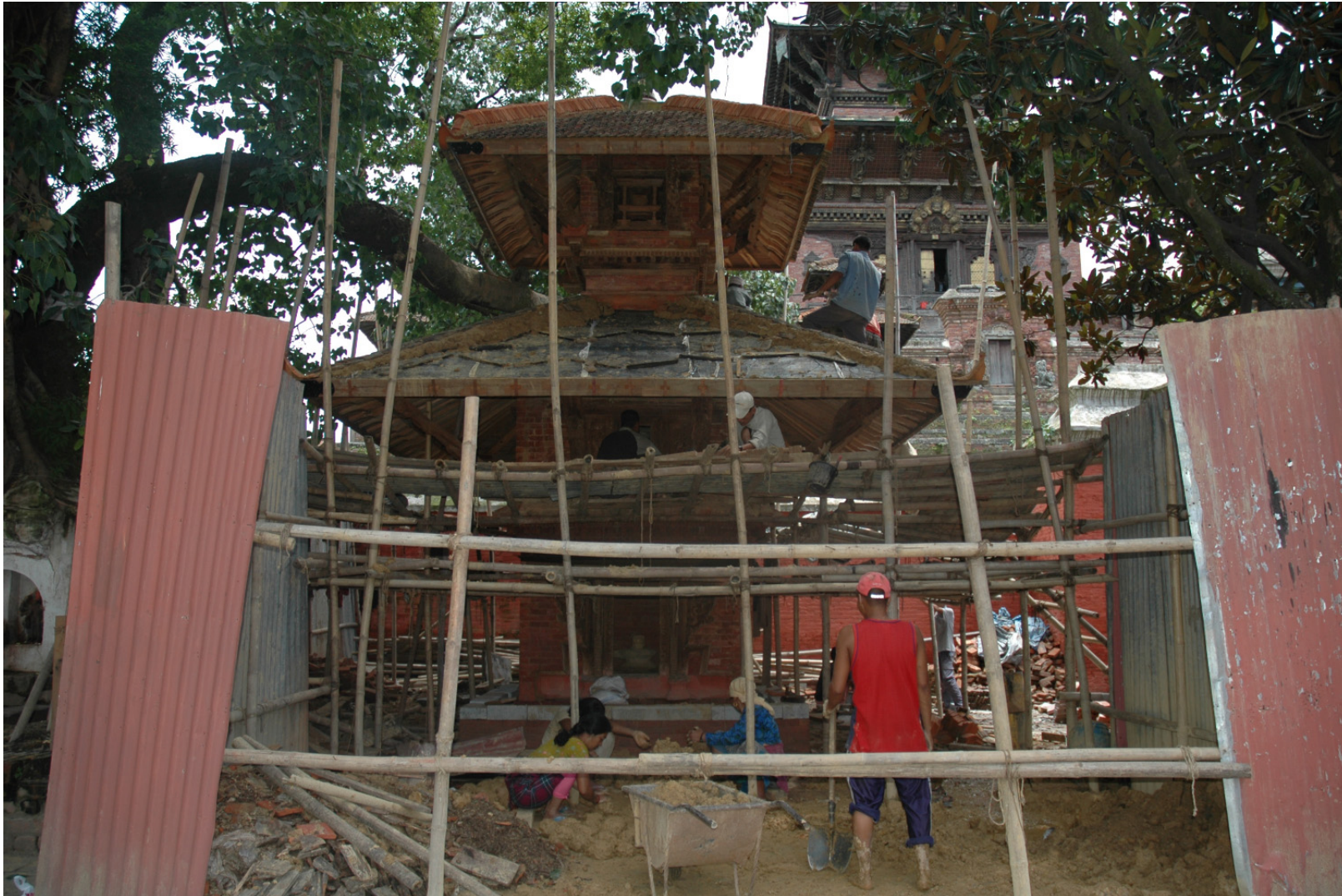
above: Battens being fixed on the roof structure to hold the mud in its position. Water proofing membrane was introduced between the planking and mud bed. Over this the traditional tiles are laid. Photo by: Lumanti Joshi, May 2007.
