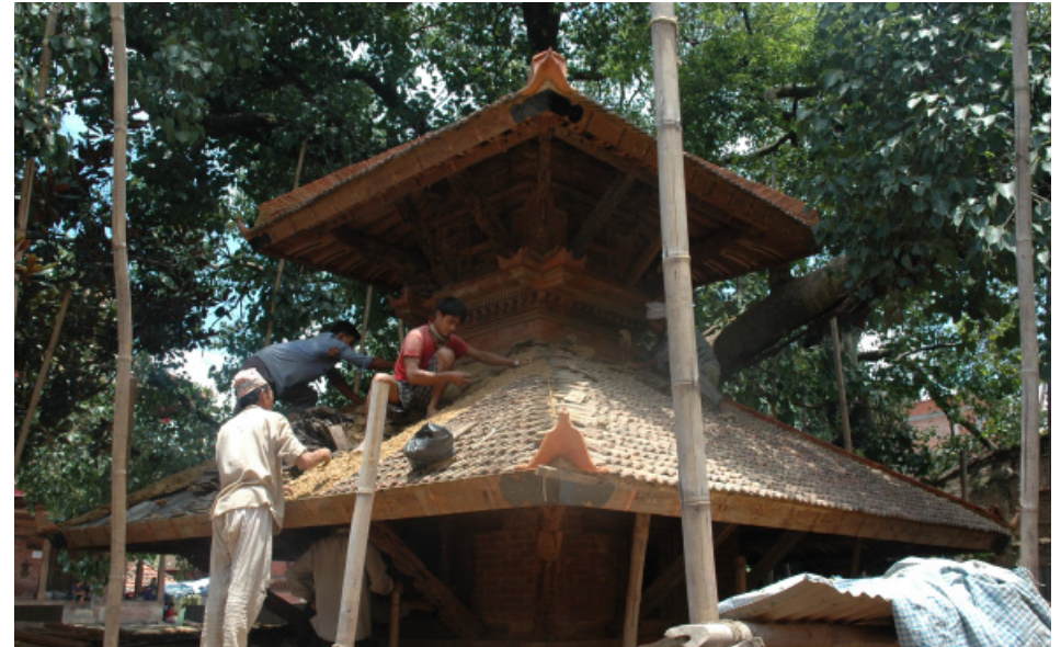
above: The masons laying traditional roof tiles on the lower roof. Photo by: Lumanti Joshi, June 2007.
