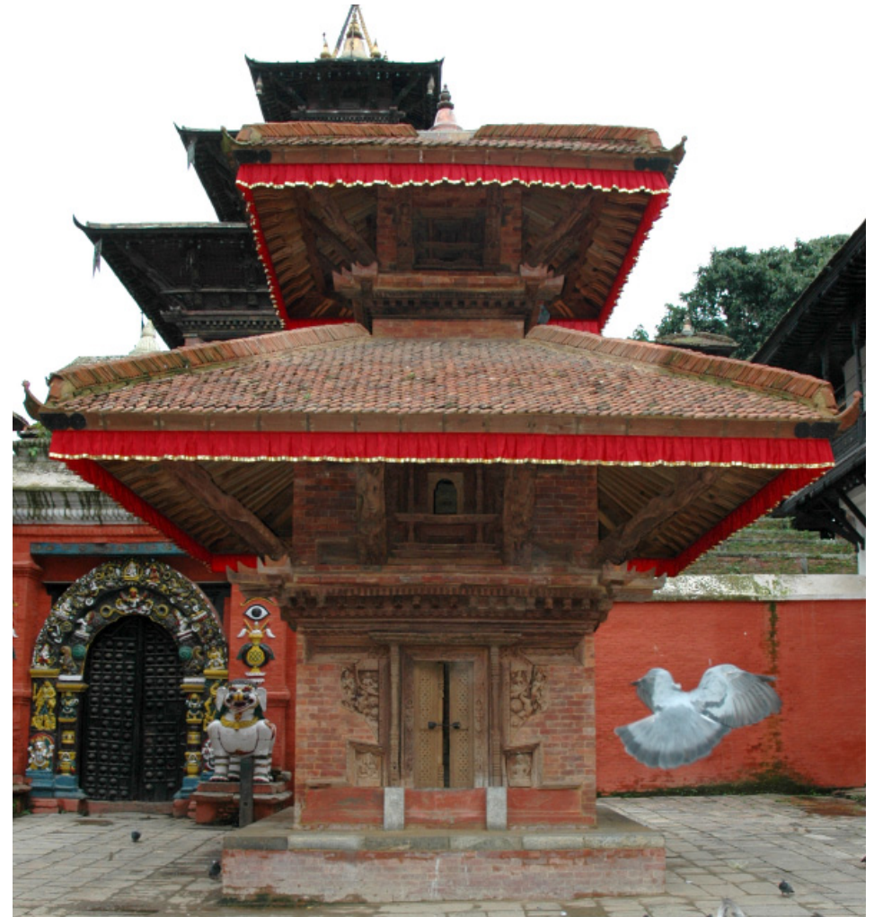
right: Mahadev Temple II after restoration. During restoration the uneven settlement of the east facade was corrected and the roof structures were also reconstructed. Photo by: Lumanti Joshi, July 2007.
