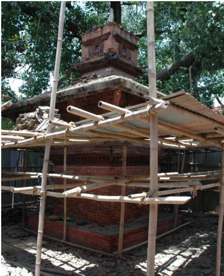
above: The upper level of the temple in the process of being dismantled. Photo by: Lumanti Joshi, April 2007.
