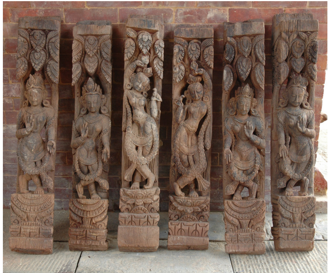
above right: The struts from both the levels were carefully brought down from their respective places, numbered and stored. The red unsightly color was removed with the help of soft brush and mild detergent, before installation. Photo by: Lumanti Joshi, April 2007.
