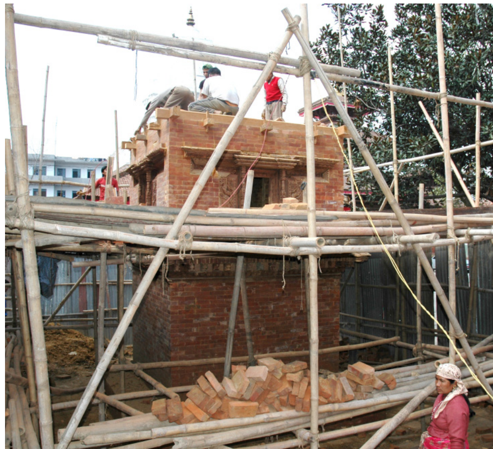
above: Construction of lower level wall being completed after correcting the settlement. Photo by: Badri Juwal, March 2007.
