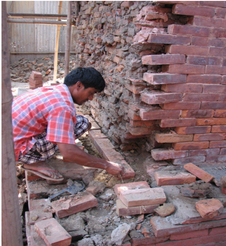
above: The lower wall being reconstructed. Damaged bricks were replaced with dachi appa set in yellow mud mortar. Photo by: Lumanti Joshi, April 2007.
