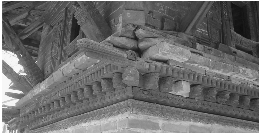
right above: New and old placed details together. Photo by: Lumanti Joshi, Dec 2006.
