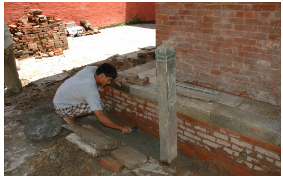
right below: Because of the poor condition of the brick work in plinth, it had to be replaced. Photo by: Lumanti Joshi, June 2007.
