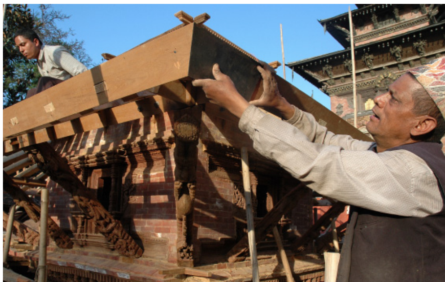
above: Construction of lower level wall being completed after correcting the settlement. Photo by: Badri Juwal, March 2007.
