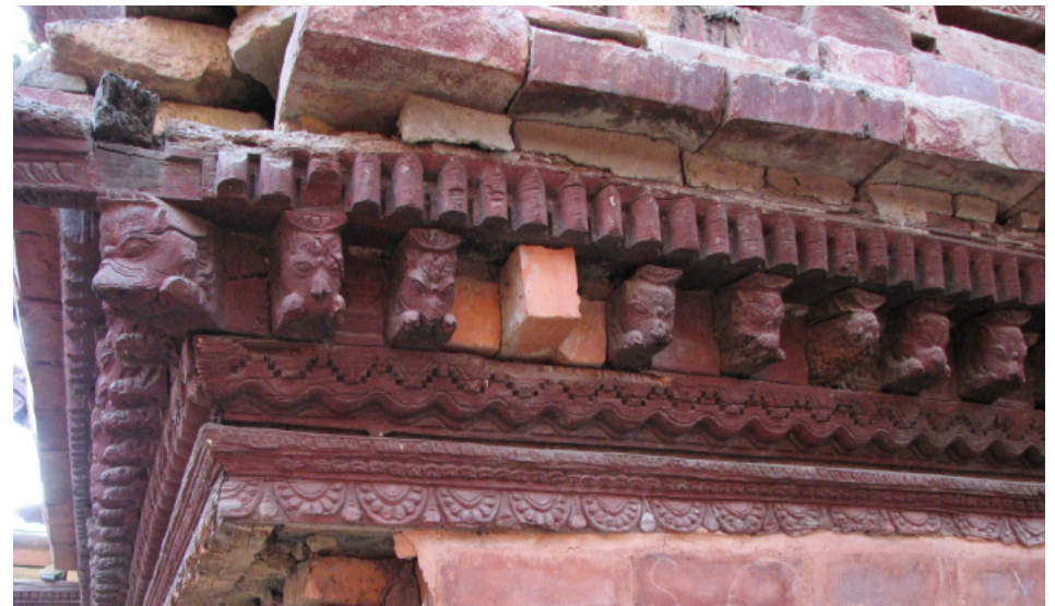
right above: The upper wall was constructed of locally available machine made bricks in cement mortar. Even the rafters were of insufficient length and had deteriorated considerably, thus could not be reused. Photo by: Lumanti Joshi, December 2006.
