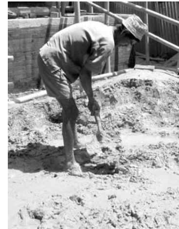
left: Kageswar Mahadev Temple with newly prepared rafters installed. A large crack developed on the parapet walls as we progressed with work, was later repaired. Photo by: Badri Juwal, KVPT, September 2005. top: Masons at work. Photo by: Badri Juwal, KVPT, May 2005. bottom left: Preparation of mud for mortar. Mud mortar construction greatly enhanced seismic performance of the building. Photo by: Raju Roka, KVPT, September 2005. bottom right: Carpenters installing the rafters. Every third rafter was bolted to the wall plate for stability of structure. Photo by: Badri Juwal, September 2005.
