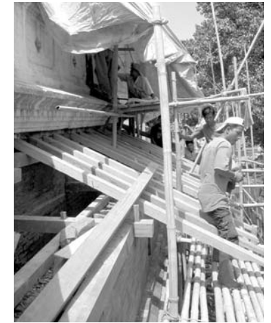
left: Kageswar Mahadev Temple with newly prepared rafters installed. A large crack developed on the parapet walls as we progressed with work, was later repaired. Photo by: Badri Juwal, KVPT, September 2005. top: Masons at work. Photo by: Badri Juwal, KVPT, May 2005. bottom left: Preparation of mud for mortar. Mud mortar construction greatly enhanced seismic performance of the building. Photo by: Raju Roka, KVPT, September 2005. bottom right: Carpenters installing the rafters. Every third rafter was bolted to the wall plate for stability of structure. Photo by: Badri Juwal, September 2005.
