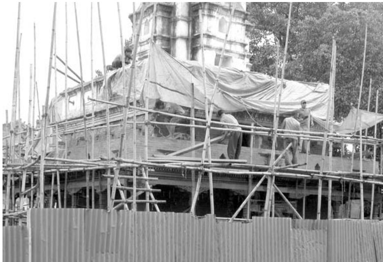
top: Damaged sections of the cornice were recarved and installed with original details. Photo by: Raju Roka, KVPT, August 2005. bottom: Walls above the beam level being rebuilt. The frame of the temple was covered with tarpulin to check the rain water seepage. Photo by: Raju Roka, September 2005. left: The roof structure was dismantled to be completely refurbished. Photo by: Raju Roka, April 2005
