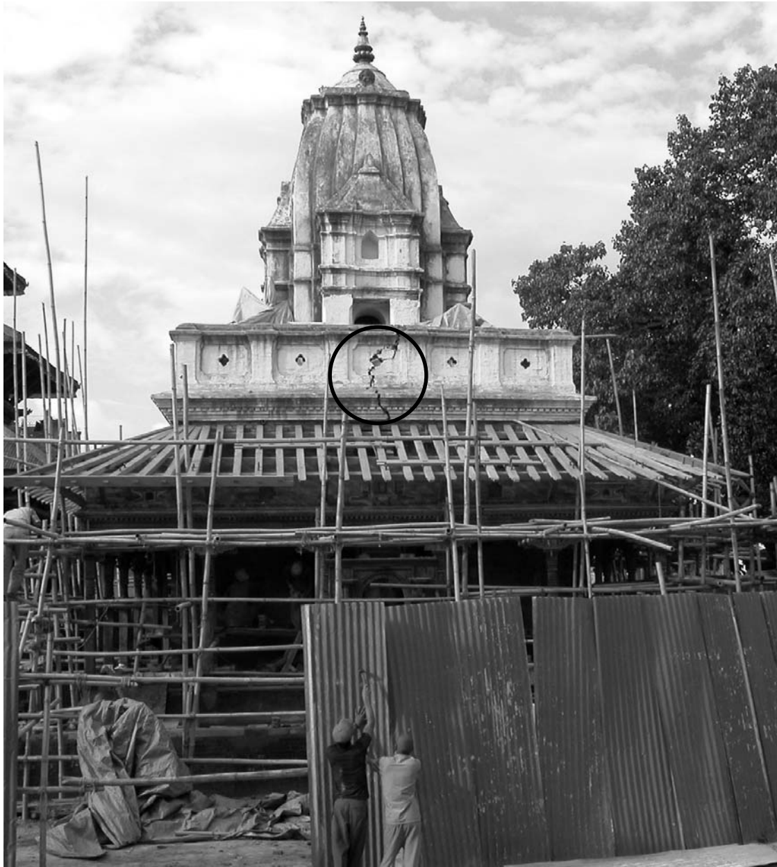
left: Kageswar Mahadev Temple with newly prepared rafters installed. A large crack developed on the parapet walls as we progressed with work, was later repaired. Photo by: Badri Juwal, KVPT, September 2005. top: Masons at work. Photo by: Badri Juwal, KVPT, May 2005. bottom left: Preparation of mud for mortar. Mud mortar construction greatly enhanced seismic performance of the building. Photo by: Raju Roka, KVPT, September 2005. bottom right: Carpenters installing the rafters. Every third rafter was bolted to the wall plate for stability of structure. Photo by: Badri Juwal, September 2005.
