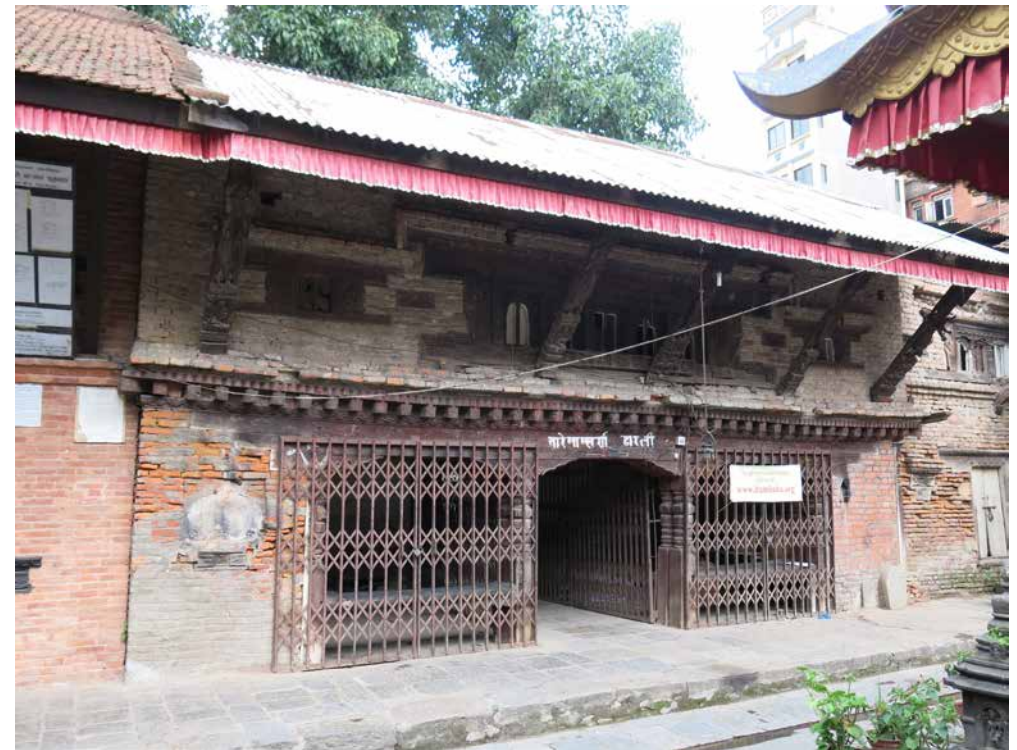
Itumbaha East Wing | 2001 Existing condition of courtyard facade before restoration.
