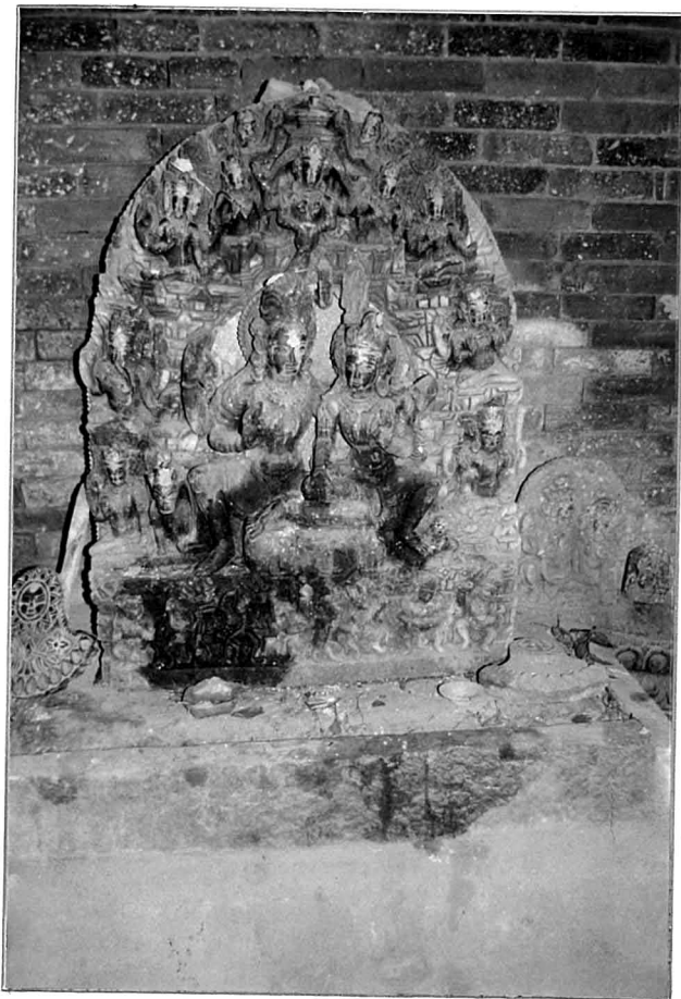
THE ICON OF UMA MAHESWAR. SALT STAINS RESULT FROM THE 1979 INTRODUCTION OF CEMENT PLASTER ON THE STONE PEDESTAL AND ANTI-THEFT MASONRY FILL BEHIND THE SCULPTURE.
