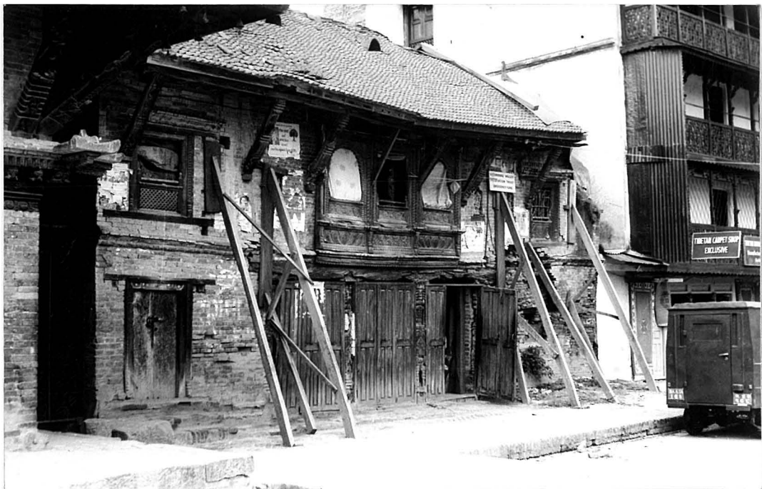
Above: multi-bay window or san jhyah of principal facade, fall, 1993. Below: principal facade spring, 1994. Notice additional wall damage at far right.
