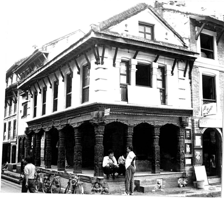
Below: Oldfield's view of Patan Darbar Square, southern end, showing the two story Lam Pati. In the distance another one story resthouse, now lost, is visible. Above: Sarasvati Pati, three buildings west of the Ayuguthi Sattal defining Patan Darbar Square. This building (rebuilt in 1989) mixes 17th c. pillars and post-1934 colonial patterns above. Opposite top: Sundhara Sattal (1700), Sundhara, a high style variation similar to constructions of the palace. Middle: sattal at Kwalkhu with fine Malla period pillars (18th century) and post-1934 earthquake superstructure. Bottom: Sattal at Uku Bahal (19th century, reconstructed 1990).
