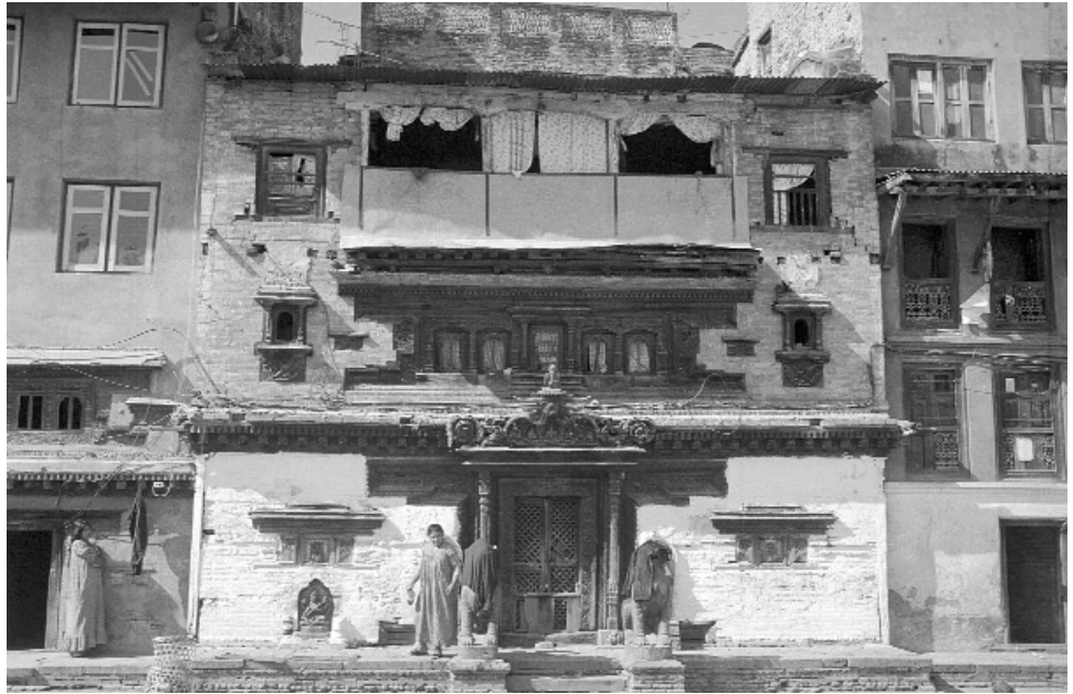
A view of shrine building before restoration in 2000. Photo: Raju Roka.
