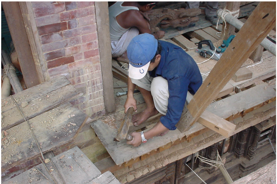
A carpenter fitting the historic corner strut. Photo: Rohit Ranjitkar, August 2002.
