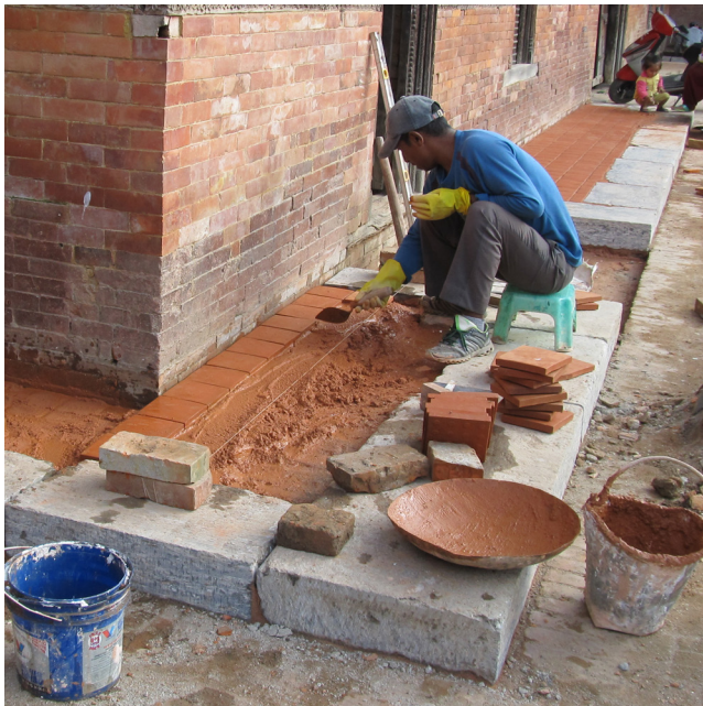
Laying tiles in surkhi mortar | October 2013 Lime and brickdust mortar was applied between the stones and on the surface of the plinth.
