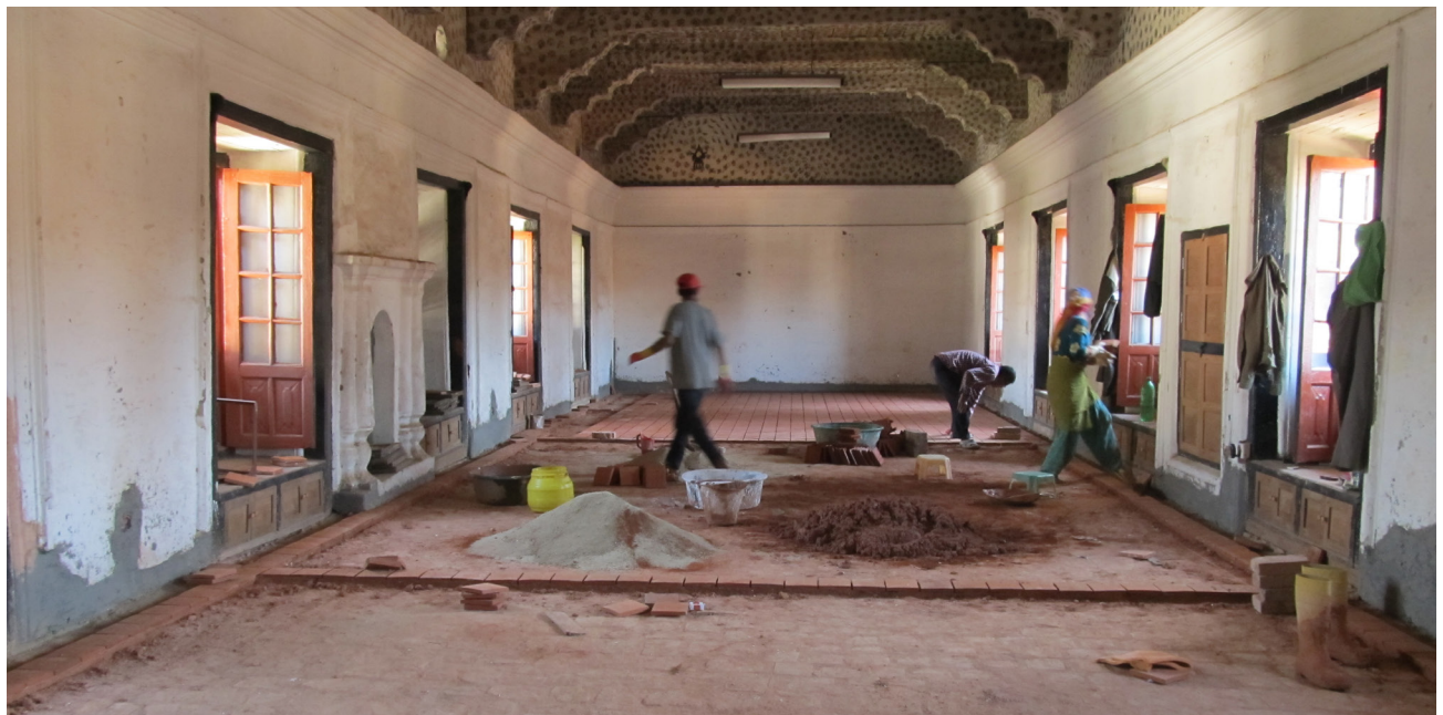
Reconstruction of the floor cover on the second floor | March 2013, November 2013 Terracotta floor tiles with lime and brickdust mortar on brick soling (bottom) were placed above a layer of plywood planking (top).
