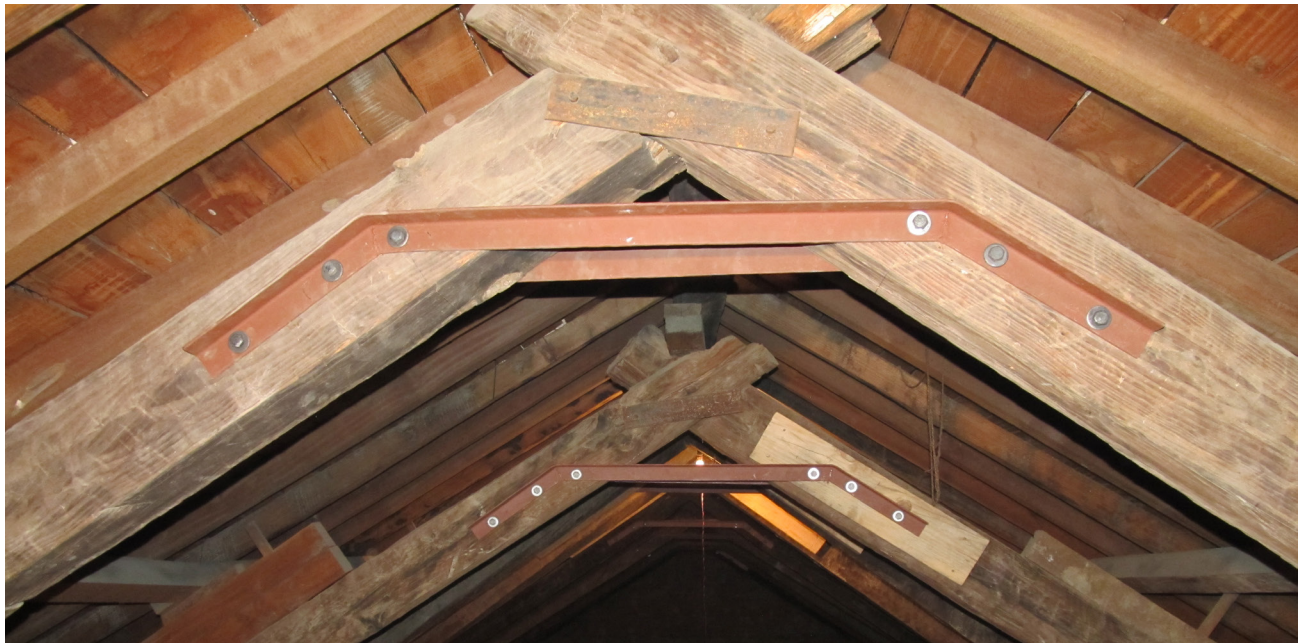
Structural reinforcement of the roof with steel collar braces | January 2014 Steel collar tie braces were firmly attached to the rafters with 1/2" bolts. This structural reinforcement will help improve the roof's resistance to seismic motion.
