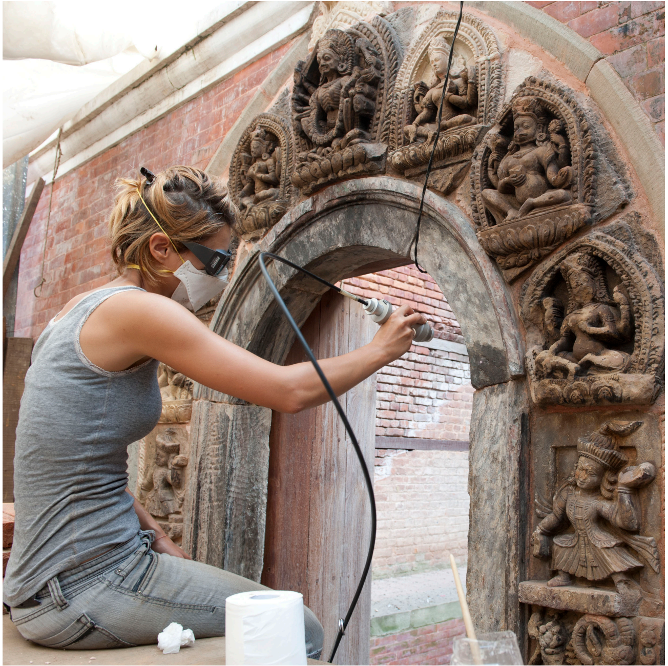
Laser ablation of tar paint | August 2013 The use of the laser enabled highly selective and targeted cleaning while avoiding surface damage.
