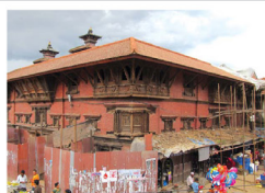
Photo taken this week during mid-restoration. A poor restoration attempt after the 1934 earthquake required entirely new roofing.
