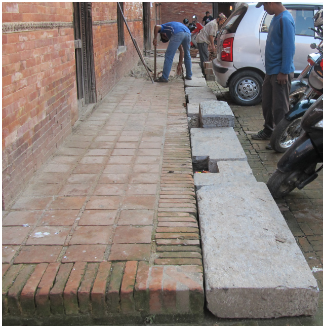
Existing condition of plinth | September 2013 New edge stones were cut to match the level of the existing plinth, consisting of tiles and on-edge bricks.
