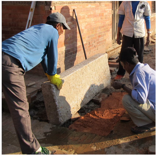
Placement of edge stone | September 2013 The plinth was dismantled and the new edge stones were laid in place on top of a bed of lime and brickdust mortar ( surkhi ).
