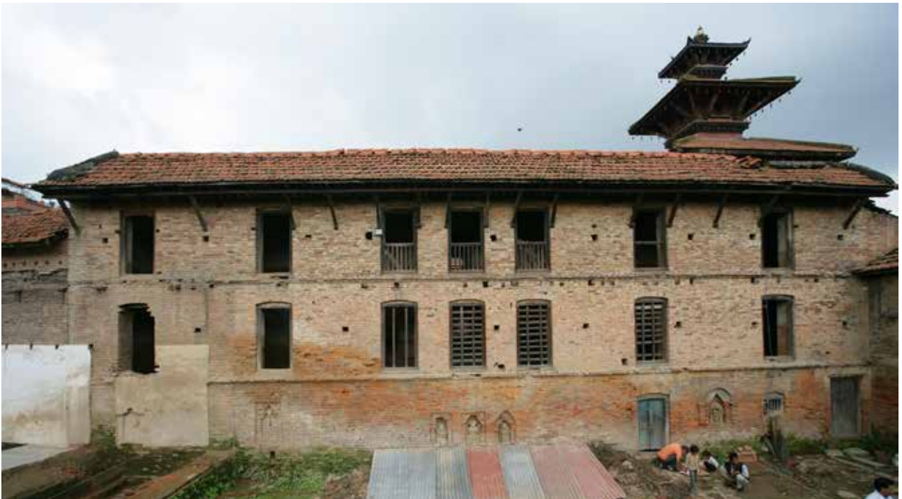
Façade facing the garden | existing condition | 2008
