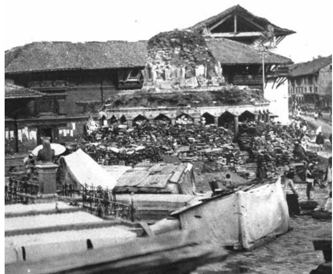
Aftermath of earthquake | 1934 The roof of the upper floor of the Court Building is visible on the far right in this photograph taken from Patan Darbar Square.
