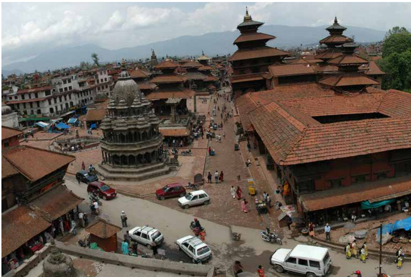
Aerial view of Patan Darbar Square with the Court Building on the right | 2006
