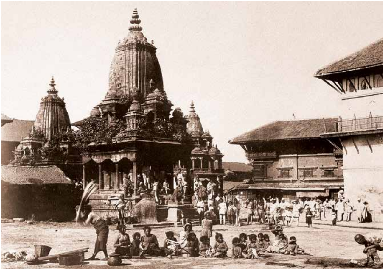
Vishweshwara Temple with the Court Building on the far right Kurt Boeck | 1899 A part of the Court Building can be seen with a timber
