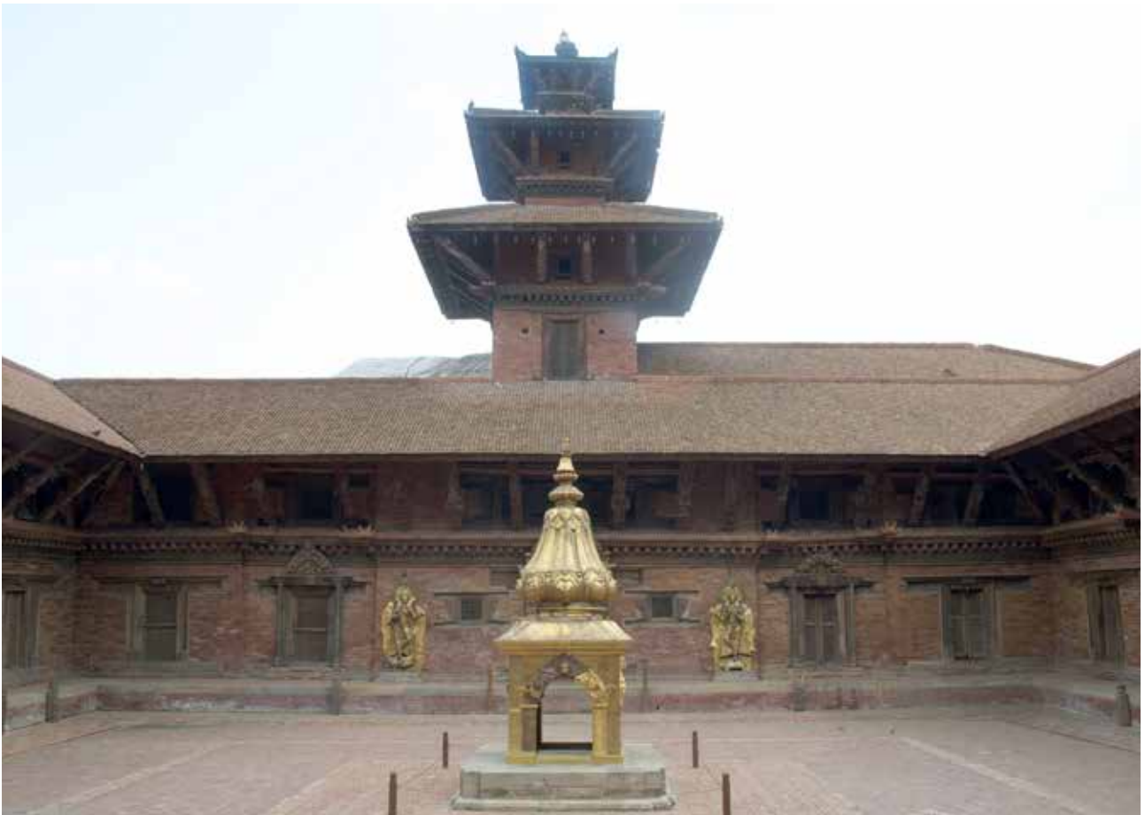
View from the North | May 2013 The South Taleju Temple towers above the roof of the Mulchowk Palace courtyard. Dasain sacrifices are carried out on the
