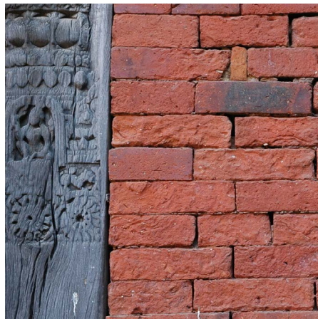
ERODED BRICK, DAMP AREA
