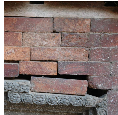
LOOSE BRICK, EFFLORESCENCE
