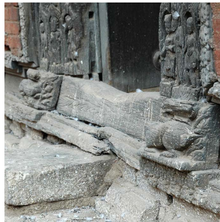
ROT, MISSING PIECE - BROKEN
