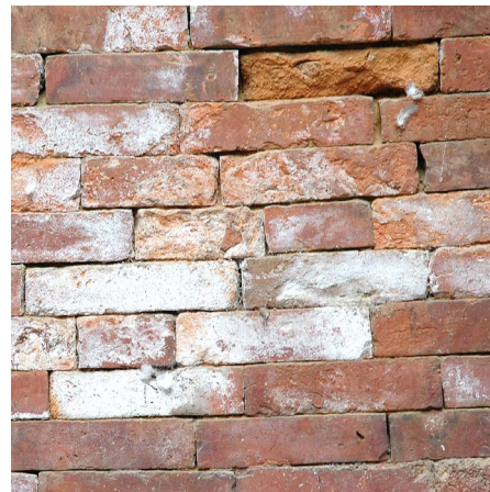
EFFLORESCENCE, SPALLING
