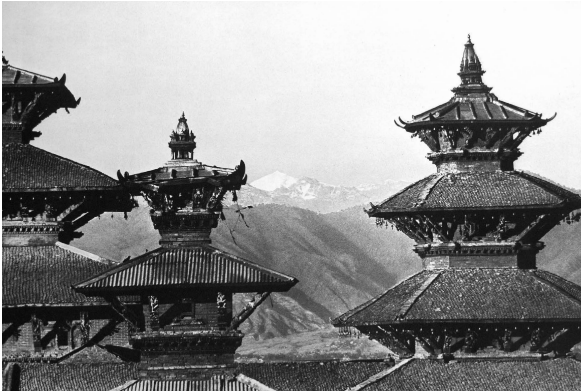
View from the south | Heinrich Seemann, 1965 The South Taleju Temple is seen here with a corrugated tin roof cover on the first and second levels. South taleju is flanked by Degutale Temple (left) and the North Taleju Temple (right) with the Langtang range in the background.
