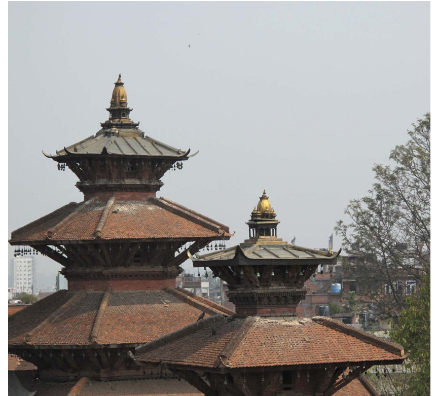
View from the south | March 2013 The South Taleju temple is seen here with the North Taleju temple in the background. The lower roof has been rebuilt with traditional terracotta roof tiles ( jinghati ) since the photo at left was taken.
