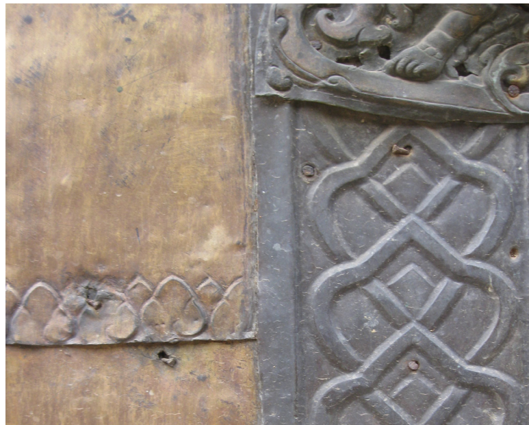
Detail of decorative frame | Nov 2011 The gilded part on the left is original, while the un-gilded part on the right is a later addition. This was affixed to the original using the crude method of fastening with nails.
