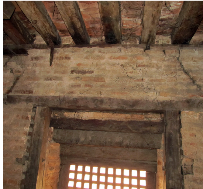
C: Crack on interior south wall | Nov. 2011 After the recent earthquake several small cracks occurred where the south wall meets the ceiling. The crack shown in the photo at left is the largest, and runs diagonally through the wall.
