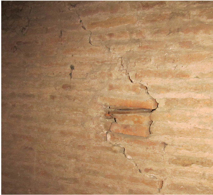
C: Crack on interior south wall | Nov. 2011 After the recent earthquake several small cracks occurred where the south wall meets the ceiling. The crack shown in the photo at left is the largest, and runs diagonally through the wall.
